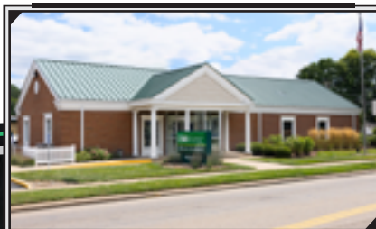
South Clay Banking Center
