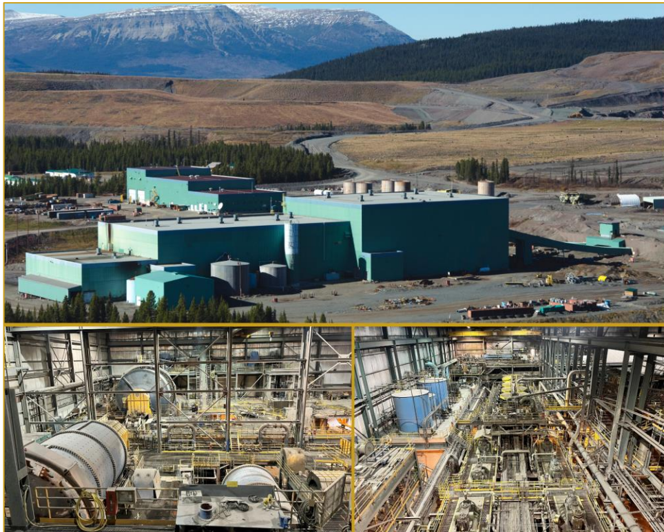
Figure 4: 50,000 tonnes per day nameplate processing plant in need of some refurbishment and equipment replacements.
