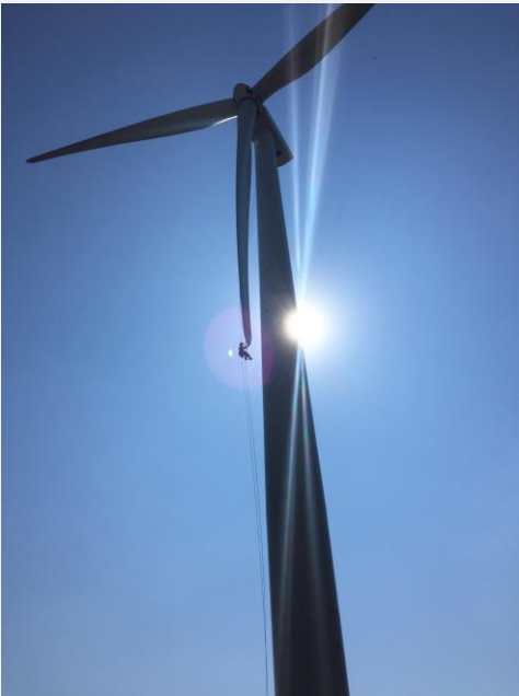
Wind turbine blade inspection and repair
