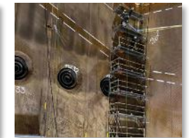
V-Deck Access Platform
