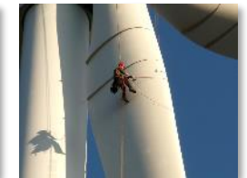
Wind Turbine Blade Inspection & Repair
