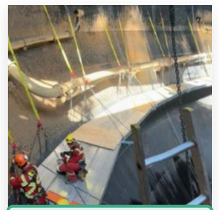
V-Deck Access Platform
