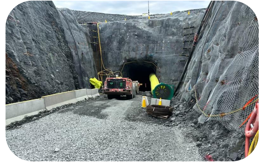
Detour Lake underground portal
