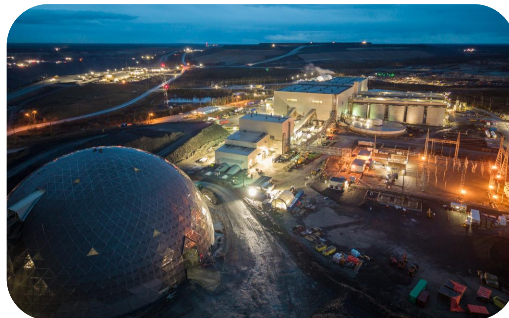
Detour Lake operations
