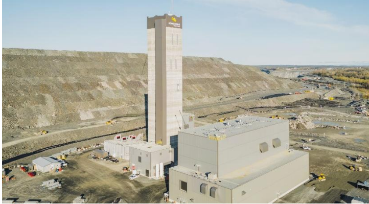
Odyssey shaft at the Canadian Malartic Complex
