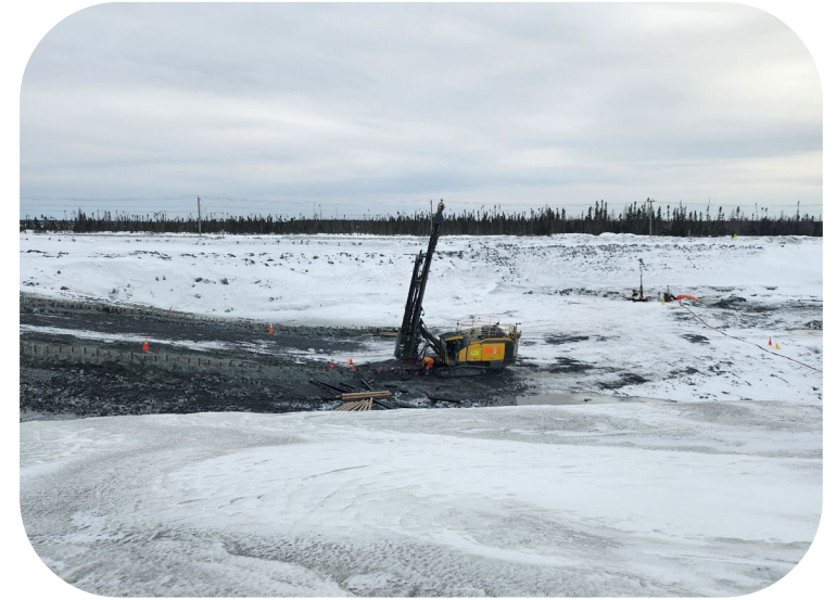
Detour Lake box-cut drilling
