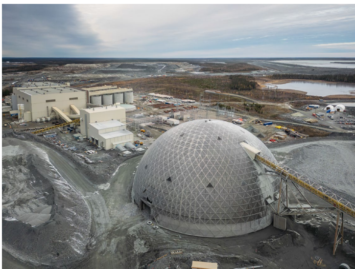
Detour Lake operations
