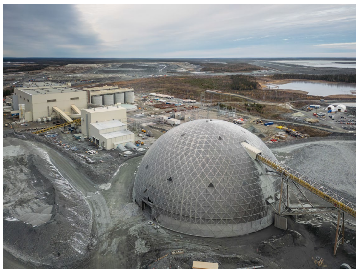
Detour Lake operations
