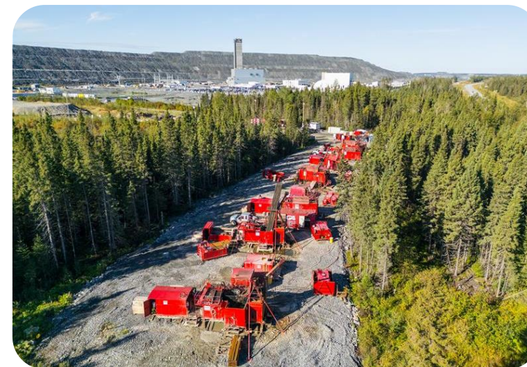
Odyssey – exploration drilling
