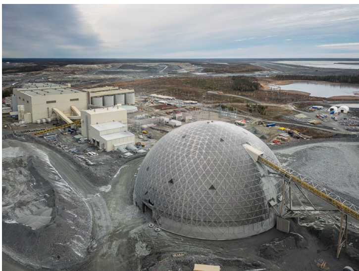
Detour Lake operations
