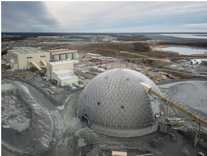
Detour Lake operations
