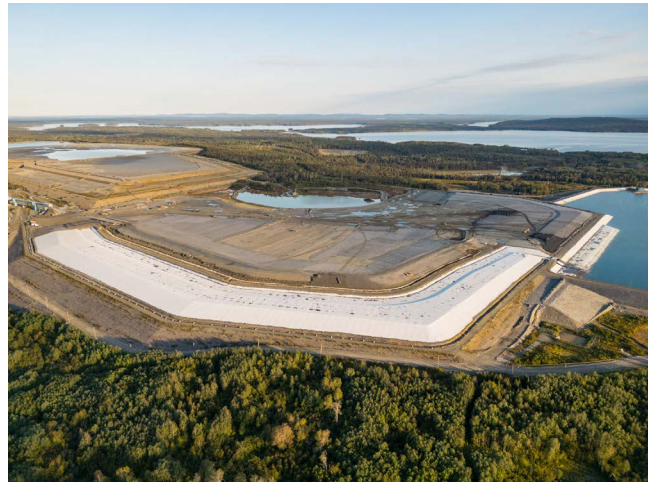
Filtered Tailings Stack constructed on a former Slurry Tailings deposition cell at Laronde, September 2024.
