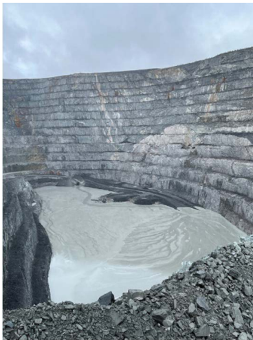
In-Pit Thickened Tailings Deposition at Canadian Malartic Mine.
