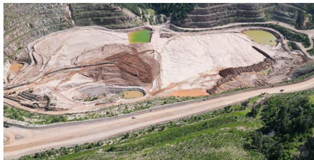
In-Pit Filtered Tailings Stack at Pinos Altos.
