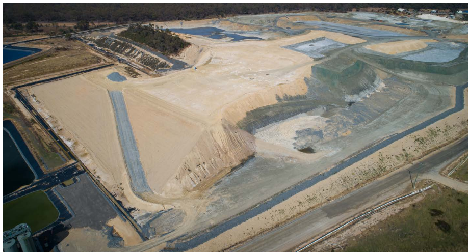
Tailings Storage Facility for one of the two streams of tailings at Fosterville.
