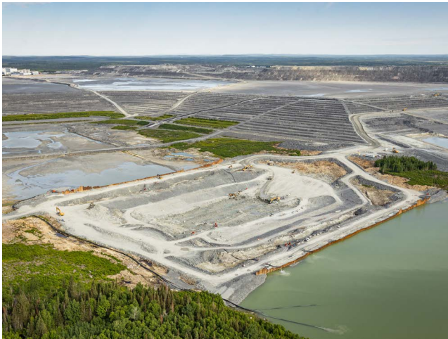
Shear Key construction at dike PR7, in 2023, at Canadian Malartic.
