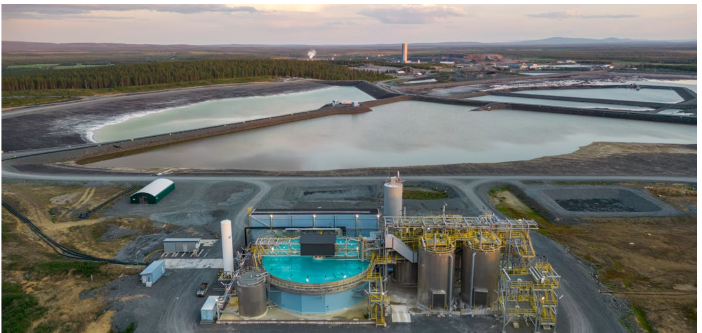
Water treatment plant at Kittilä (Lapland, Finland).
