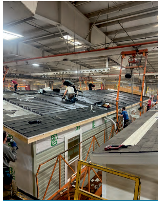
INSTALLATION OF SOLAR SHINGLES AT CHAMPION HOMES, INC. FACTORY IN PARTNERSHIP WITH GAF ENERGY
