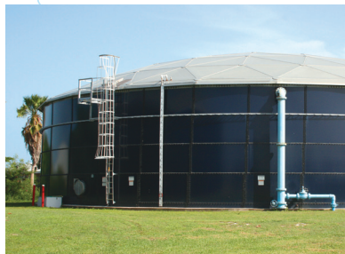
1 million U.S. gallon finished water storage tank located at our West Bay plant Grand Cayman, Cayman Islands
